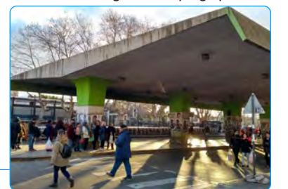
Quilmes Intermodal Station
