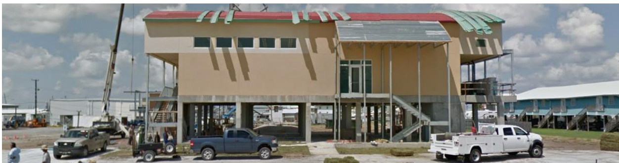
Figure 2. Government facility in Port Fourchon, Louisiana (image courtesy of Google).
